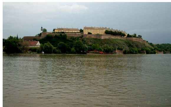
Fig. 3 Petrovaradin Fortress (“The Gibraltar of the Danube”) one of the many fortresses along the Danube River in Serbia. They were engineered as defensive outposts, for navigation security and border patrolling between empires. The cornerstone was laid in 1692 by Charles Eugène de Croÿ (photo by A. Hegediš).
