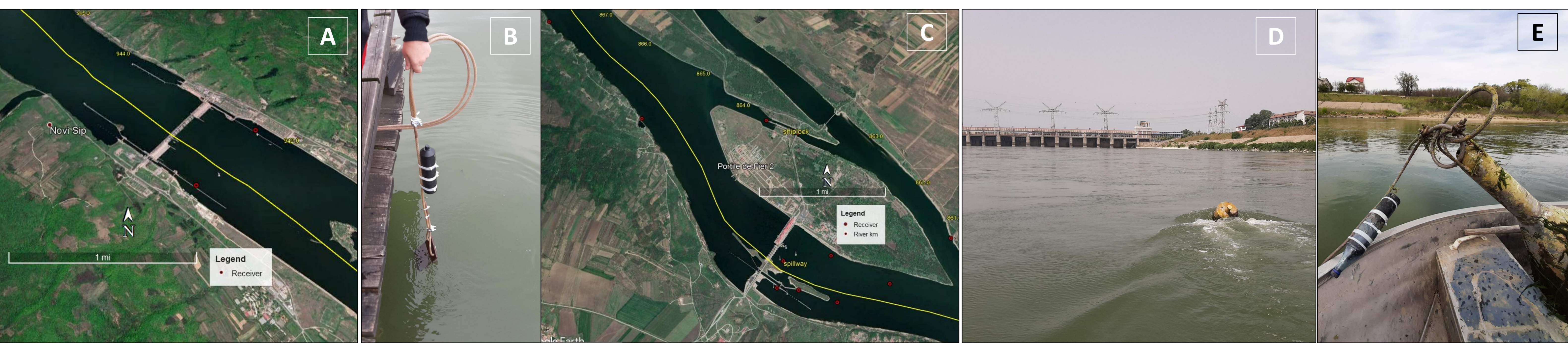
(A)-Receivers installed at the Iron gate I, attached to the concrete walls of the power plant on the right bank of the Danube River in Serbia and on the left bank in Romania; (B)-Receiver installed at the Iron gate II, upstream Romanian ship locks; (C)- Receivers location at the Iron Gate II; (D) & (E) Receivers installed downstream Iron Gate II main turbines, during the retrieval for downloading the data;
